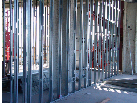
Figure 1: Framing of typical interior partition (photo by E. Miranda).
