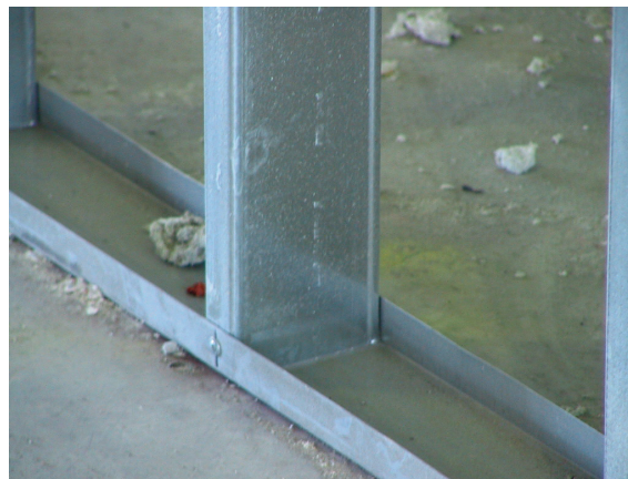
Figure 3: Photo of typical connection between stud and lower track (photo by E. Miranda).
