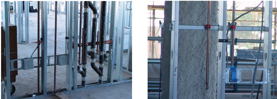
Figure 2: Examples of plumbing and electrical installation in gypsum wallboard partitions (photos by E. Miranda).
